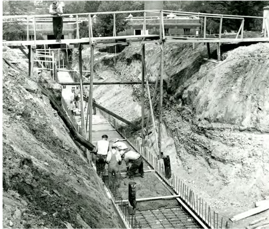
Expanding the steam tunnels
