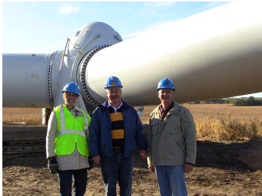
Installing a wind turbine (2011)
